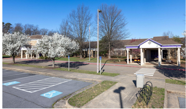
Stone Spring Elementary School 1575 Peach Grove Avenue Harrisonburg, VA 22801
